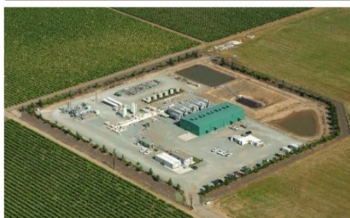
Installations Lodi et Kirby Hills
